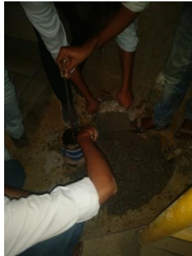
Figure 7: Casting of Cylinders
