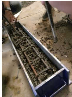
Figure 5: Casting of Beams
